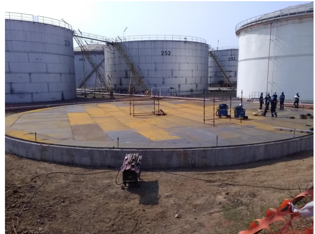
Example // SAMCOL - BP/TOTAL Terminal Expansion (Mozambique)
