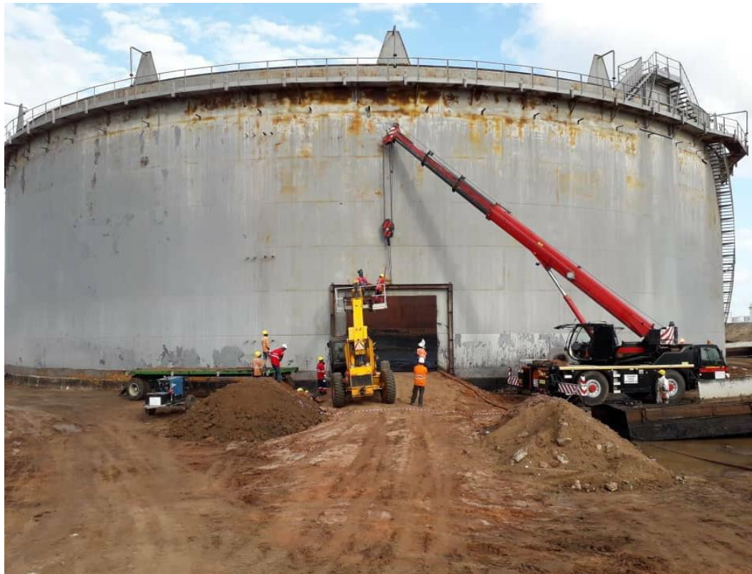
Example // TIPER Terminal Expansion and Revamping (Tanzania)
